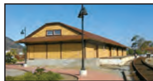
SLO's restored Historic Freight House and the SLO Railroad Museum's new display track which will be dedicated on Saturday.
